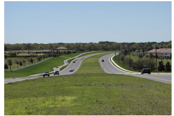
CR 486 in Citrus County provides regional connection between SR-44 and US-41 as well as providing trail and pedestrian facilities. In order to meet future travel demand, additional lanes can be accommodated in the center median.
