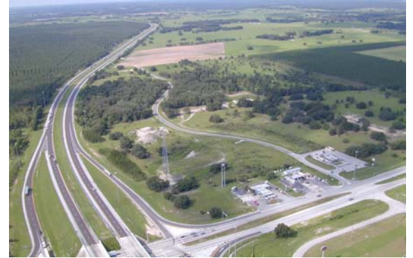
Expanding the capacity of I-75 in Hernando County is an important regional priority and will provide enhanced connectivity with other regional markets.
