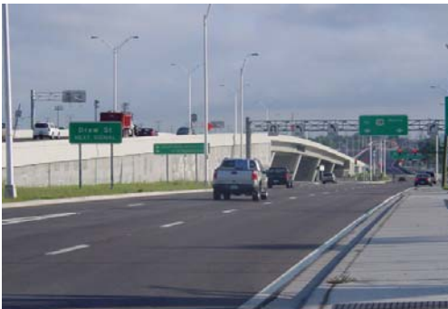
U.S. Highway 19 is the backbone of Pinellas County's regional transportation network and one of the CCC's top priorities. Interchanges such as this at Drew Street in Clearwater are a key strategy in meeting mobility needs in the corridor.
